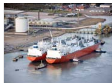
Figure 2: Dockside high-pressure gas transfer systems are thus far the most common type of standby terminal. Photo courtesy of Exceleerate Enerav.
